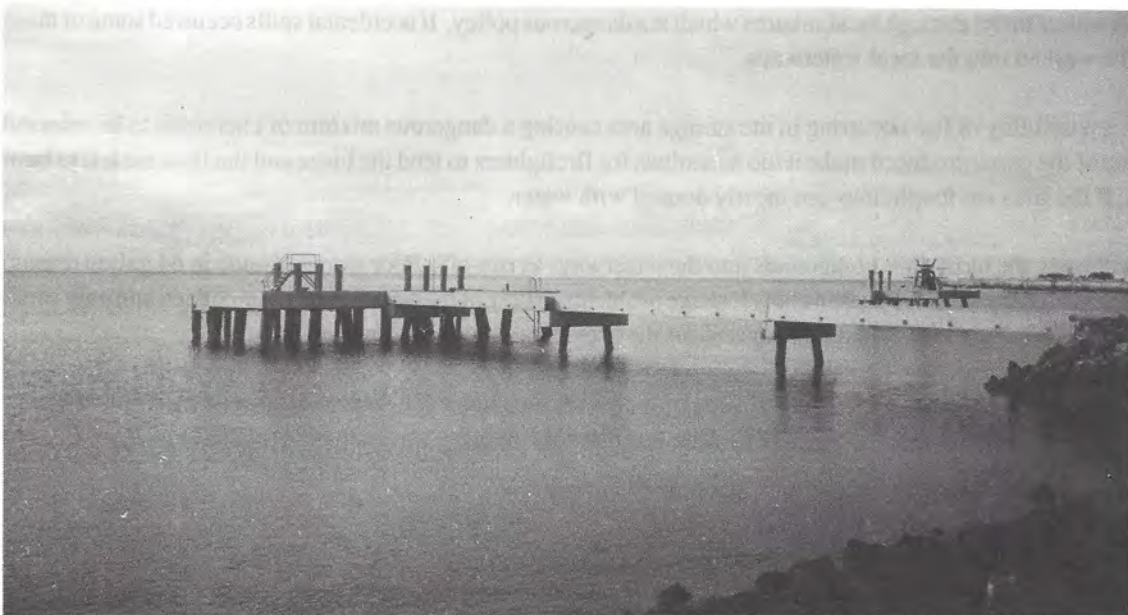
Fig 2.13: In an effort to give large ships access to land many piers are being built. This new pier is being build on Fisherman Island, Brisbane.
