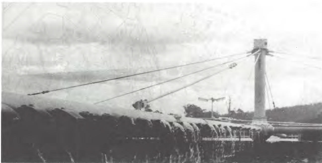
Fig 3.12: Trickle filter aeration (secondary treatment).
