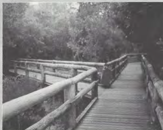
Fig 3.46: Elevated walkways have been built to allow public access to beaches without destroying the natural vegetation.
