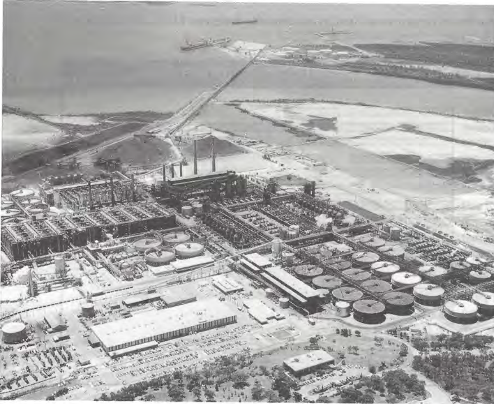
Fig 3.32: Alumina processing plant. (Photo courtesy Queensland Alumina)
