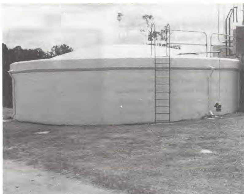
Fig 3.44: A digester which is used to produce biogas.
